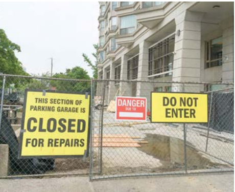
Ongoing construction in Momiji’s front parking lot. (Photo by Momiji Staff.)
